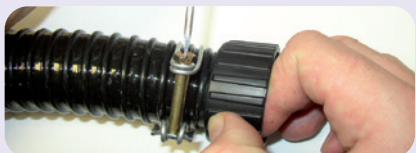
Tighten up clip to make it watertight
